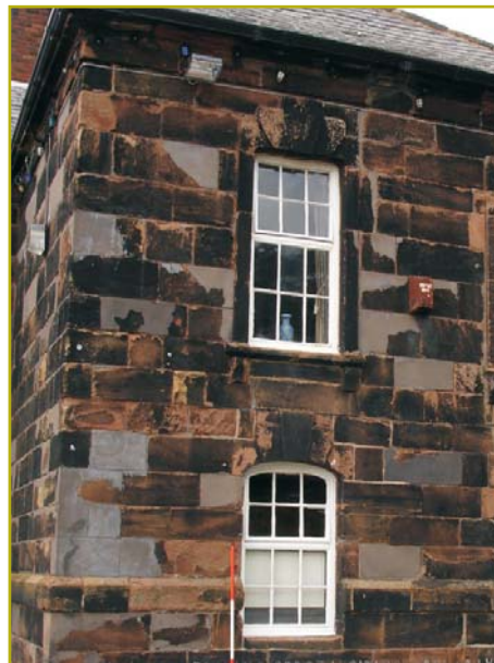
Figure 34: Examples of hard cement mortar damaging stonework: (above) Hard cementitious mortar joints damaging a stone boundary wall and (right) Damaging and unattractive cementitious render repairs
