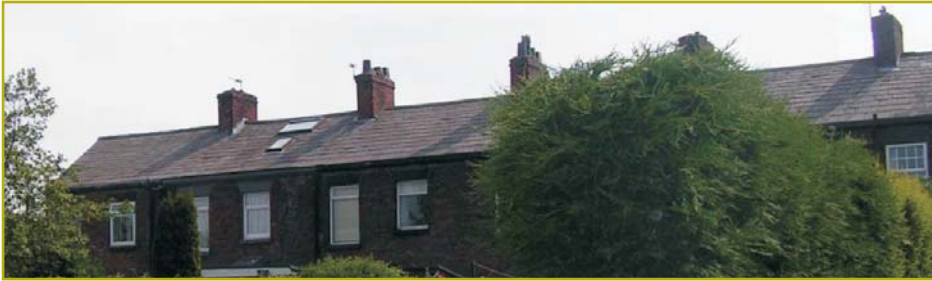
Figure 33: The effect of rooflights on the roofscape of a row of terraced housing
