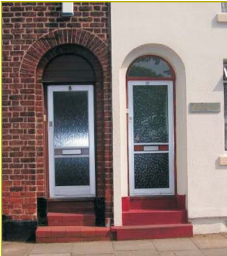
Figure 31: The effects of replacement doors on the character of buildings in Halton Village
