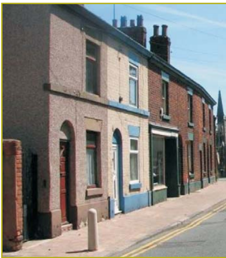
Figure 36: The effects of stone cladding and pebbledashing on individual housing and the overall street scene
