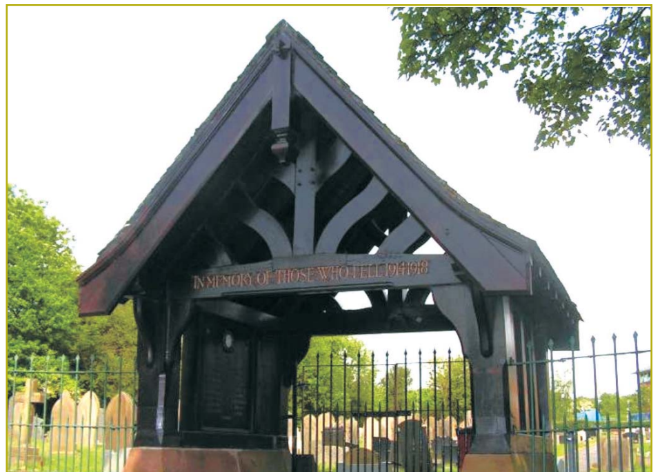
Figure 18a: Lych Gate marking the entrance to Halton Cemetery from Holt Lane
