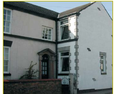
Figure 30: The effects of replacement UPVC windows on the character of buildings in the Conservation Area
