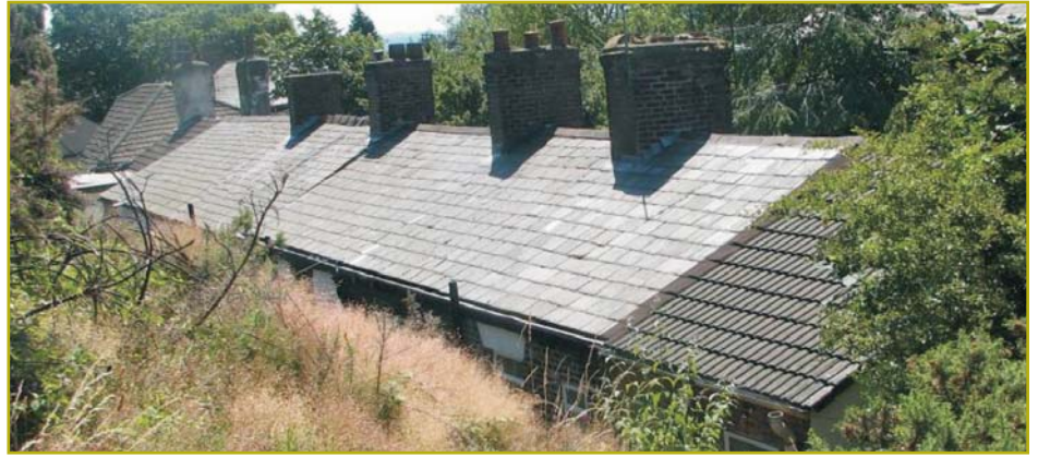
Figure 32: The effects of replacement roofs on the character of the village's roofscape
