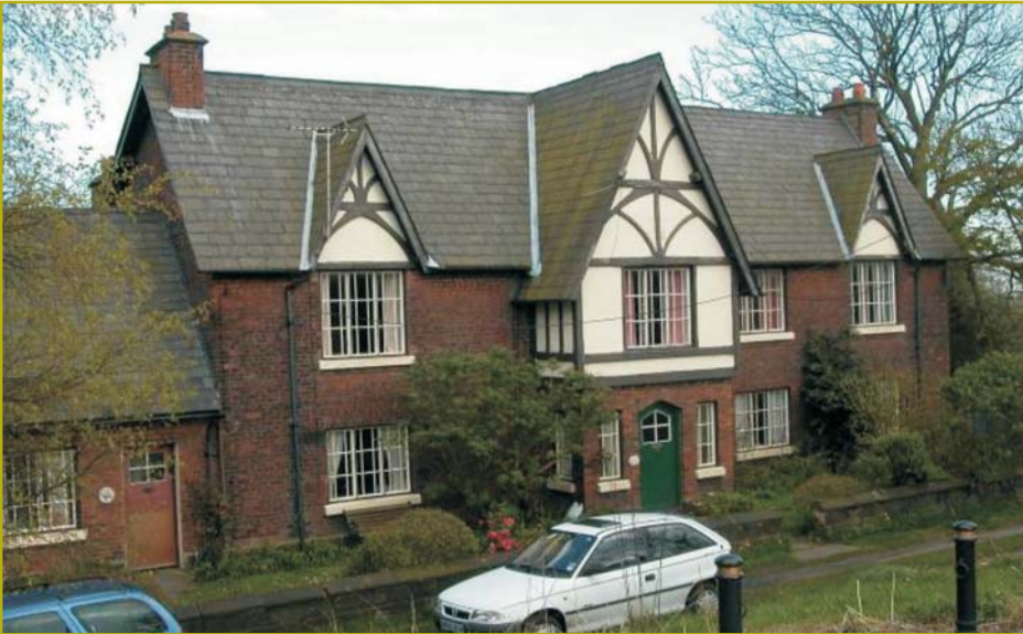
Figure 2 1b: Hill House, Castle Road
